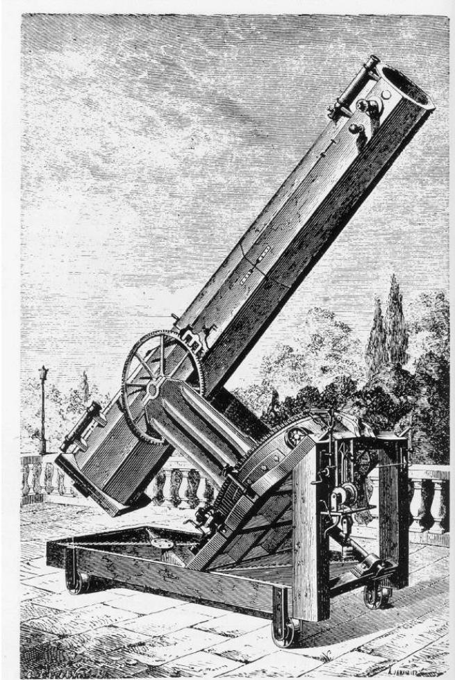
Fig. 5.8. Foucault's largest (80 cm) silver-on-glass reflector, completed in 1862 (reproduced from King [5.2])
