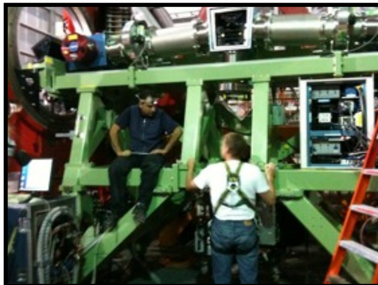
Completing the electrical system
